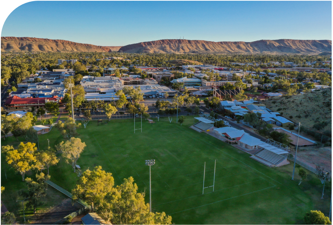
Alice Springs Township aerial photo
