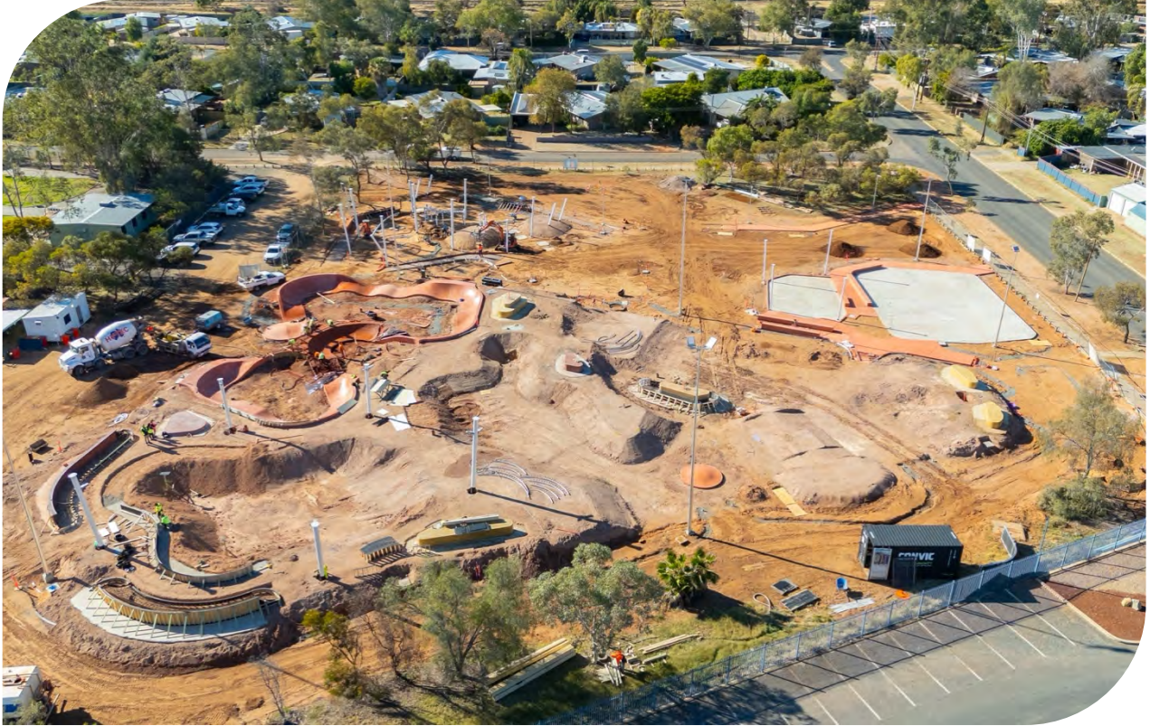
Newland Park works in progress, aerial photograph 2025
