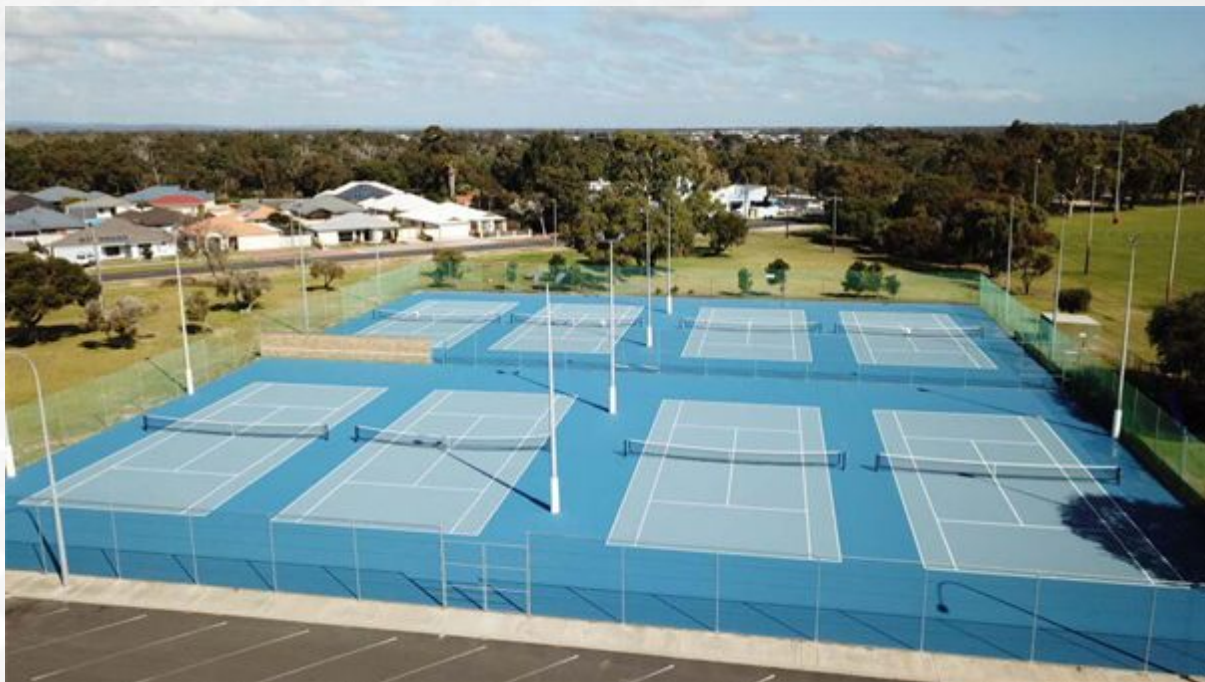
8 Laykold Masters Float on cracked asphalt bases
