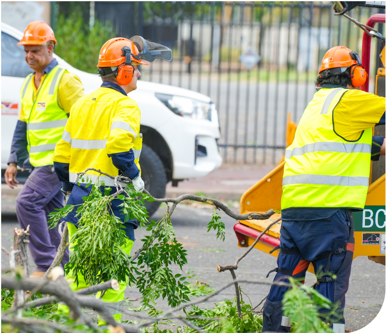
Depot team members cleaning up after severe weather
